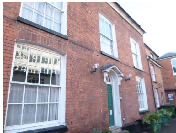
Fig.7: 21a King Street, adjoining the meeting house (just visible to the right)
