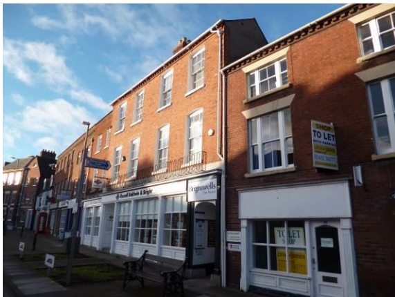
Fig.6: north side of King Street and the passageway to the meeting house (centre)
