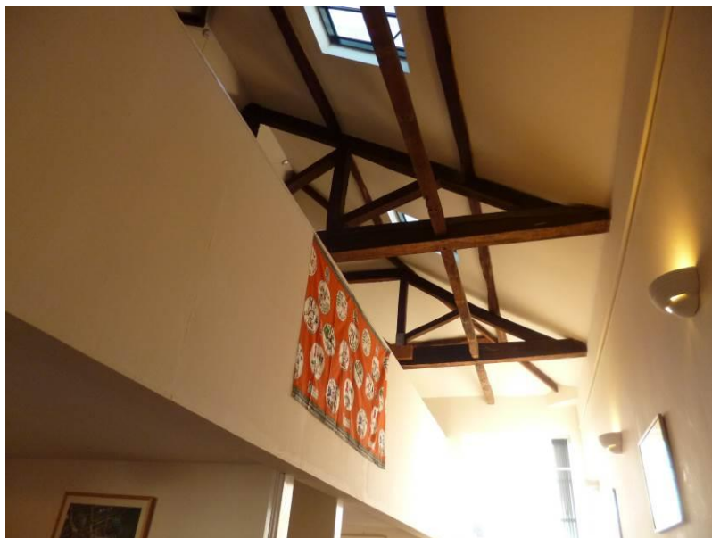
Fig.2: exposed roof in south range, from east (in office use)
